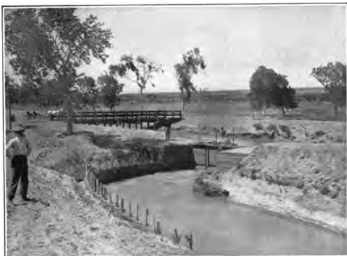
WOODEN HEADGATE OF LATERAL WITH BRUSH BANK PROTECTION. This prevents erosion and silting of channel at down points.
